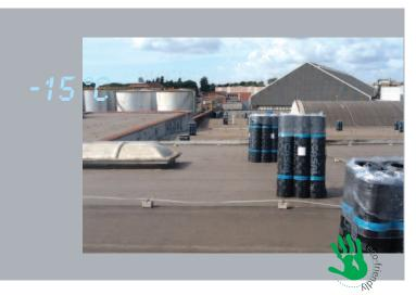
**PROJECT SPECIFICATIONS:** polyolefin polymer APP compound suitable for exposed multilayer systems with self-protected finish, painted or under heavy protection; finishing element in multi-layer systems and for waterproofing projects used with bituminous waterproofing membranes of the Enduring Quality range.
